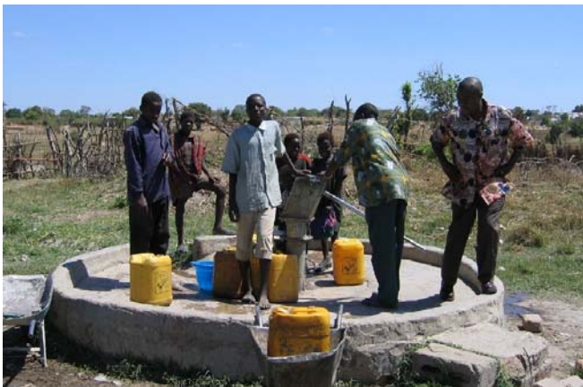
Pump equipped borehole in Zambia
