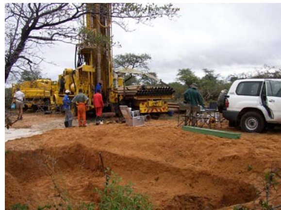
Drilling rig and down-hole borehole geophysical logging in Namibia
